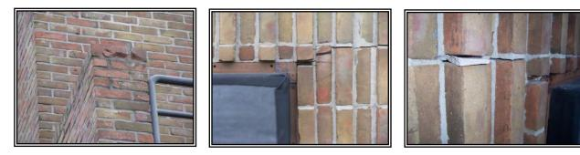
b. Some signs of efflorescence on the brick on the south and west elevation of the Training Tower which indicates some water penetration. This may be taken care of at the same time the tuck pointing repairs are made.
